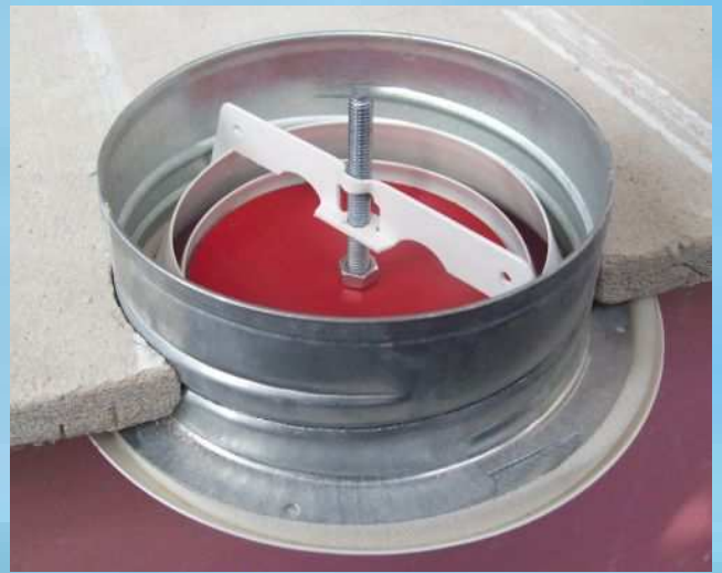
Fire Rated Ceiling Air Valve installed before a fire
